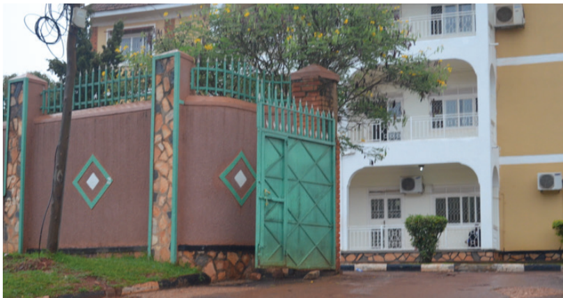
Photo 2: The Inaccessible Nakawa High Court Premises before it was closed. The premises didn't have ramps to enable the disabled access it.
